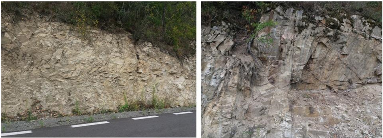
FIGURE 3 Outcrops with basement formations on the southwestern part of the Țicău mountains ( O_1 and O_2 in Figure 2). [Colour figure can be viewed at wileyonlinelibrary.com ]
